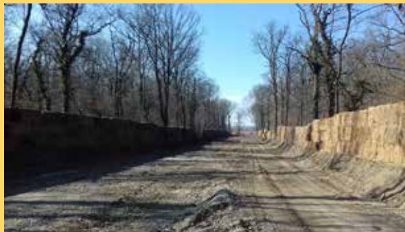
Modrone Forest: opening of the path and positioning noise barriers
